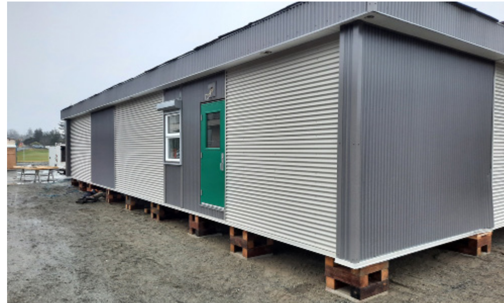
New Build at Forest Park
